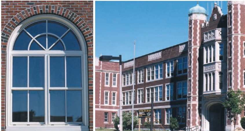
Graham replaced all the windows in East Boston High School, in the shadow of Logan Field, with special acoustical windows that shut out air traffic noise from classrooms overlooking the busy airport.
