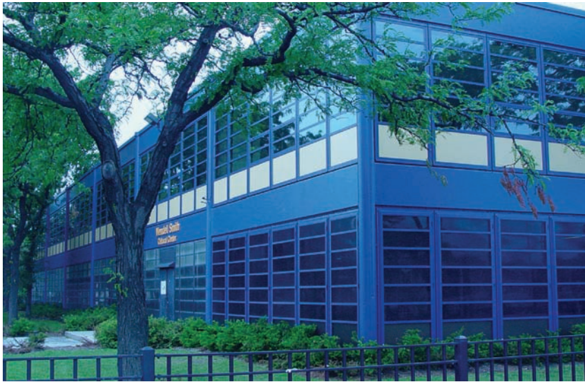
Graham school windows help control the sun with low-e glazing, internal blinds, and multiple operating systems for good ventilation. (Shown: Lincoln High School, Denver.)
